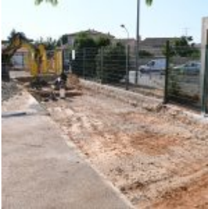
Ecole maternelle Jacques Brel – Travaux (2)
