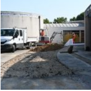
Ecole maternelle Jacques Brel – Travaux (1)
