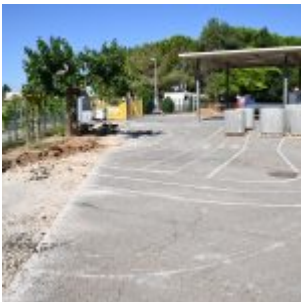
Ecole maternelle Jacques Brel – Travaux (4)
