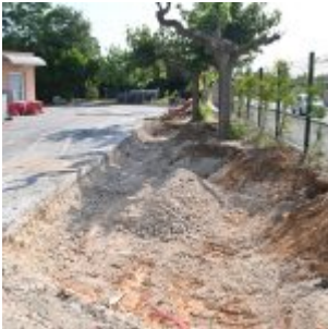
Ecole maternelle Jacques Brel – Travaux (3)
